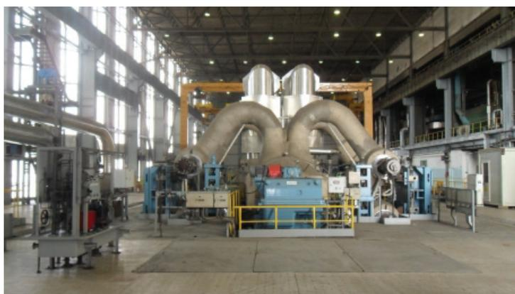
Figure1 - Block TPPKO B2 steam turbine, 350MW
